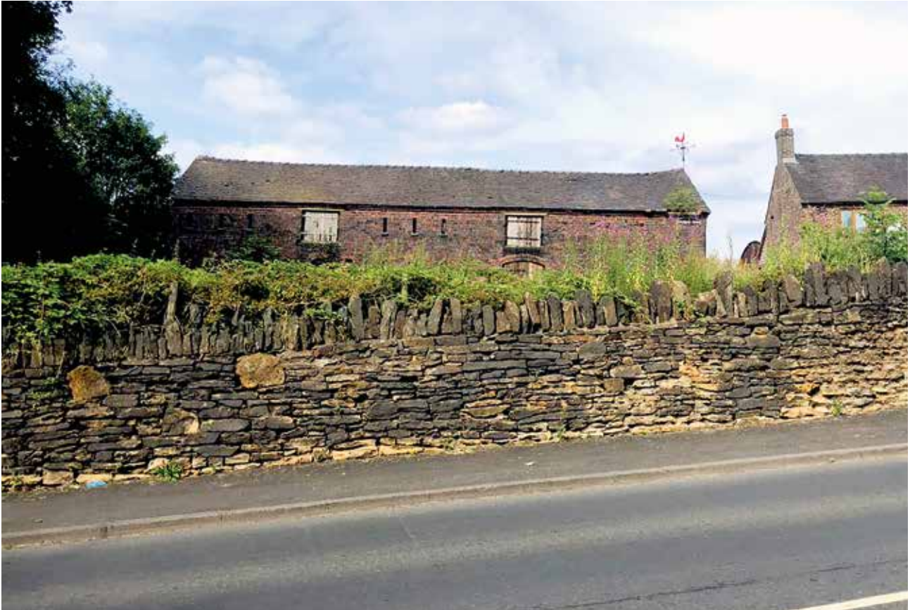
Figure 5.15, Example of heritage stone wall and farm buildings at Alsagers Bank
