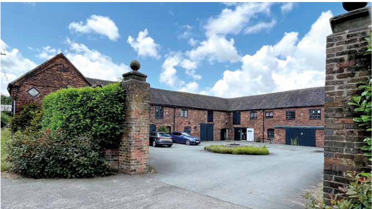
Figure 4.4, Converted farm buildings into small business units at Townhouse Farm, Alsager Road, Audley
