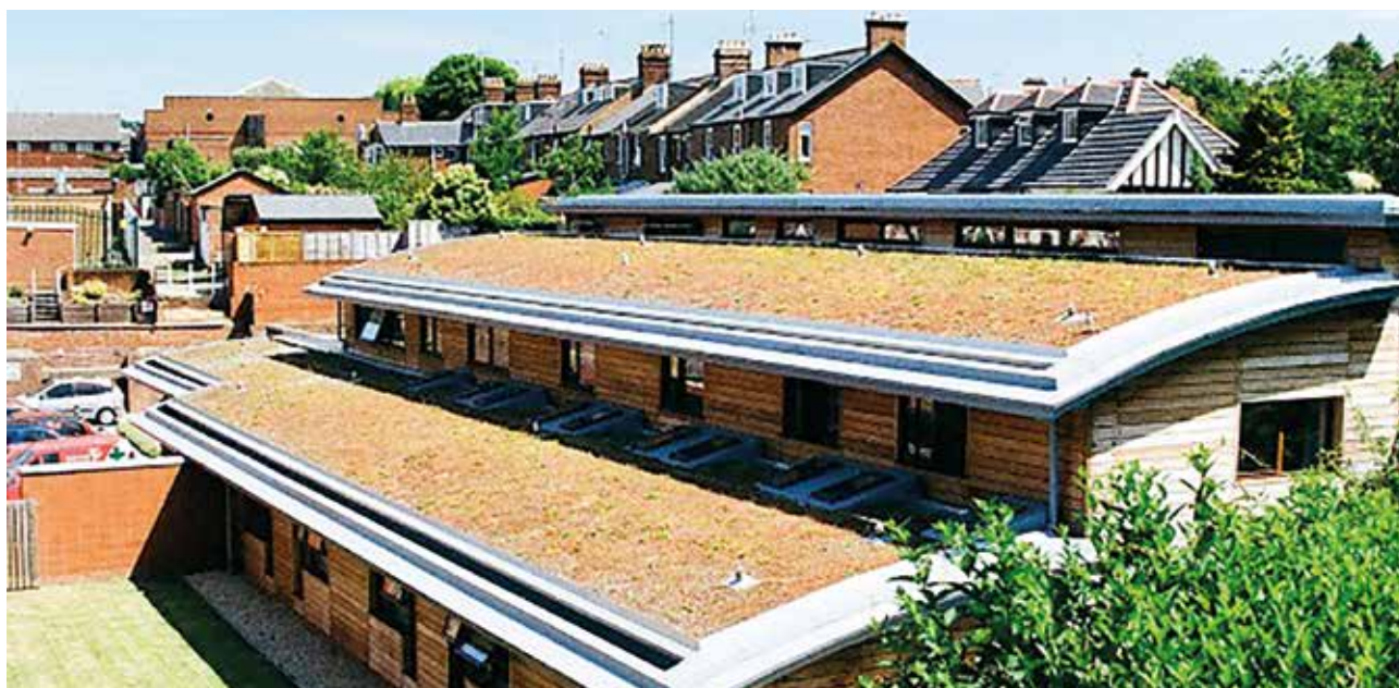
Figure 8.2, Example of green roof on a community building
