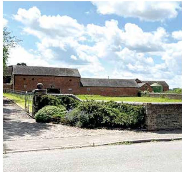
Figure 5.2, Staffordshire farmstead example at Wall Farm, Nantwich Road, Audley
