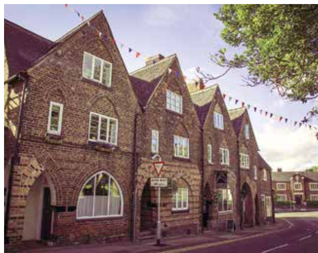
Figure 3.2, The Arches, Church Street, in Audley conservation area
