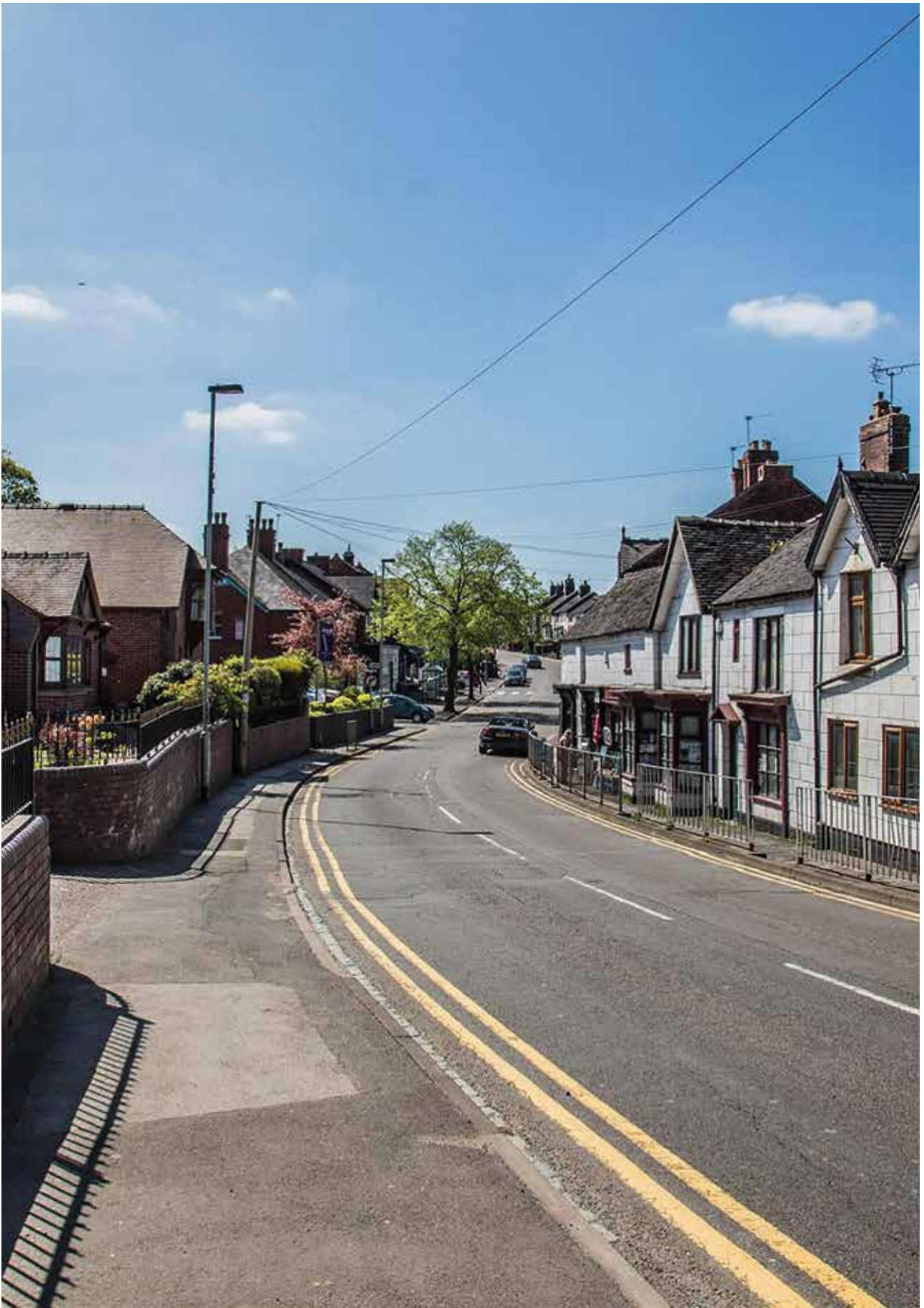
Figure 5.16, Mix of Shopfronts and Housing within the Conservation area in Church Street, Audley
