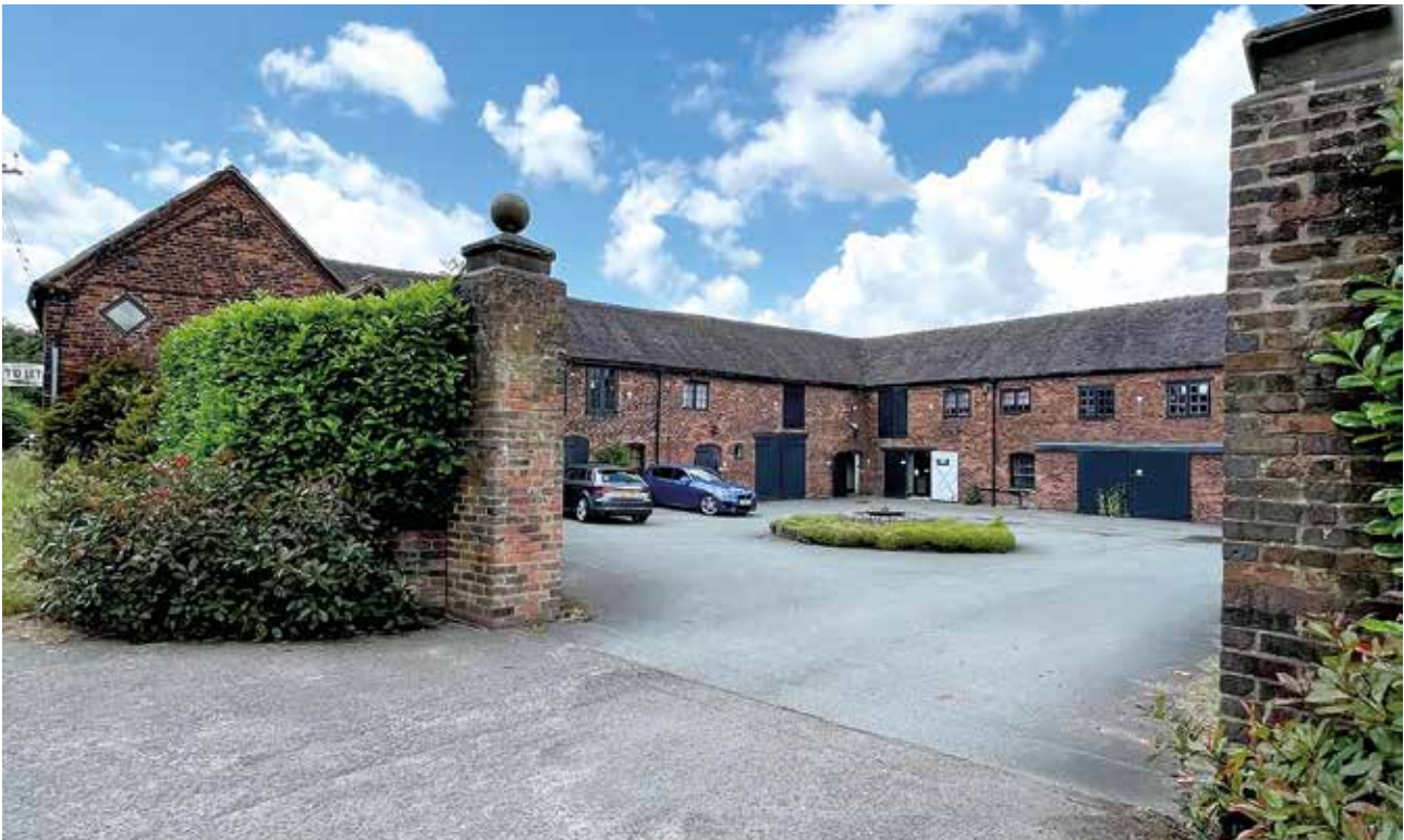
Figure 4.5, Converted farm buildings into small business units at Townhouse Farm, Alsager Road, Audley
