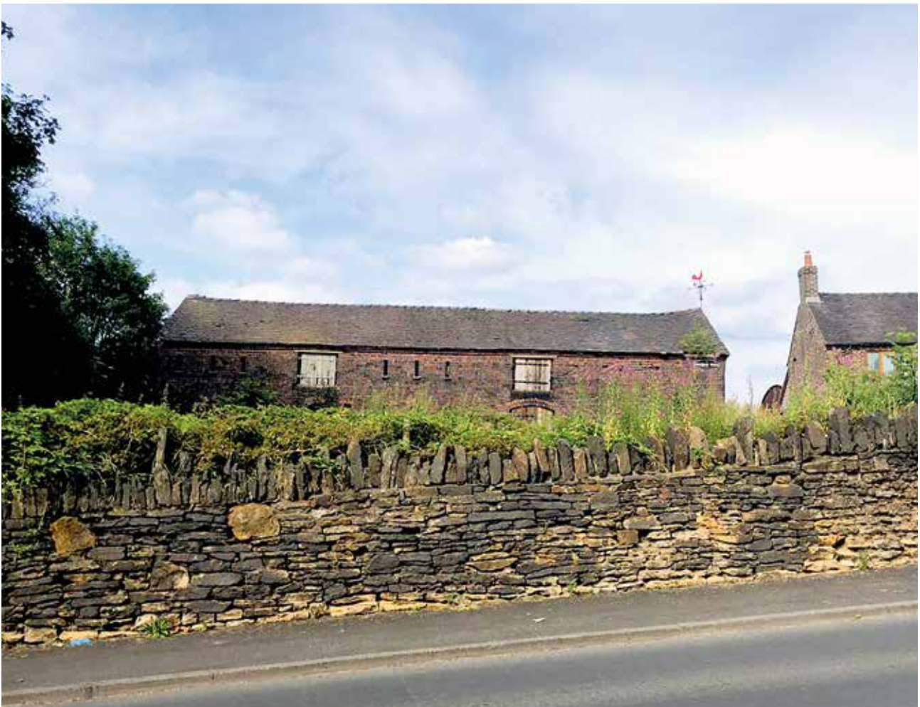
Figure 5.13, Example of heritage stone wall and farm buildings at Alsagers Bank
