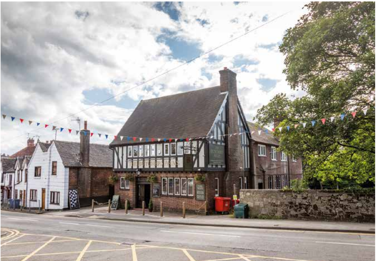
Figure 5.12, Audley Conservation Area, Church Street
