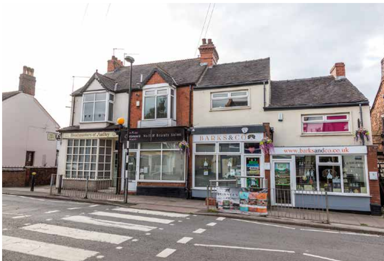
Figure 5.15, Shopfronts in Church Street, Audley
