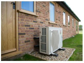
**Figure 165:** Air source heat pump unit located to the rear / side elevation of a dwelling, so to avoid its visual impact on the dwellings frontage and wider streetscape
